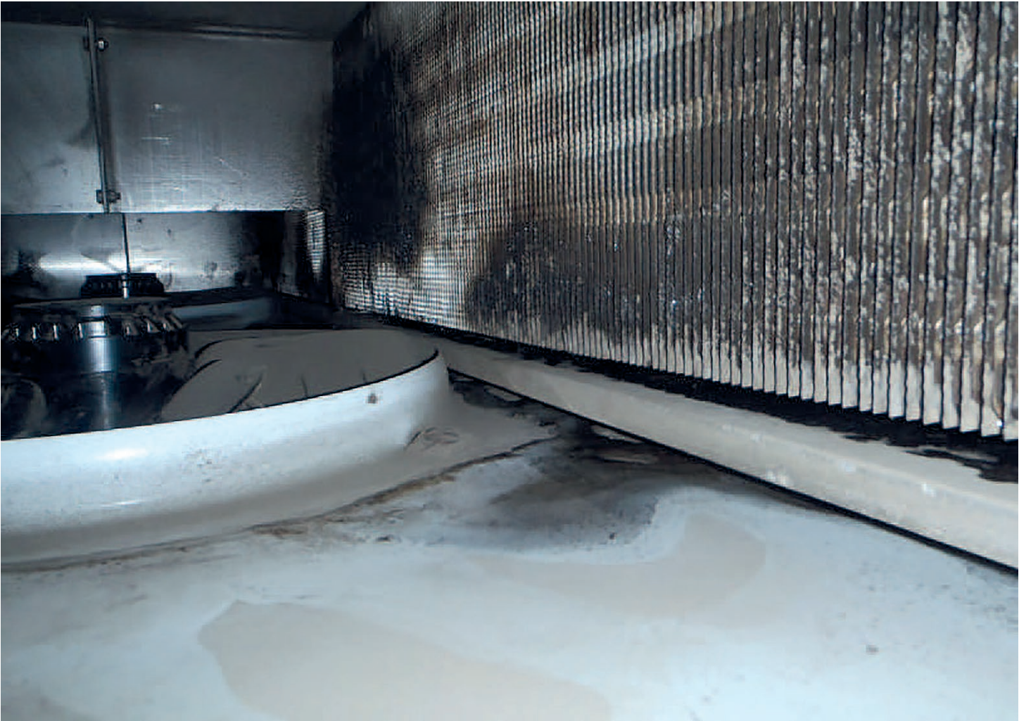
Inside Dual Discharge Cooler: Dark Area shows where wash down is required
